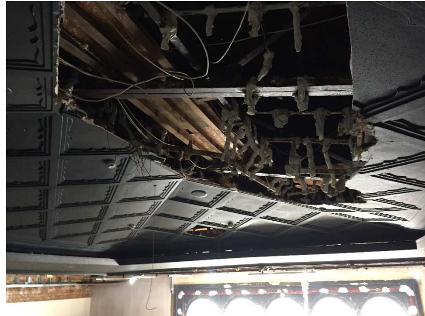
Existing suspended ceiling and roof frame
